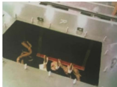
Photo 1. View of the inside of the tank through the handhole
