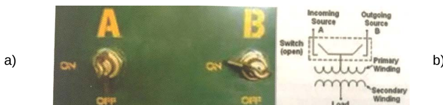
Figure 9.4 a) Loop Feed Switch b) Schematic of the Loop Feed Switch.
